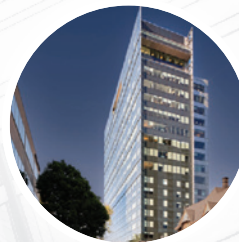
Broadway Tower Portland, OR
